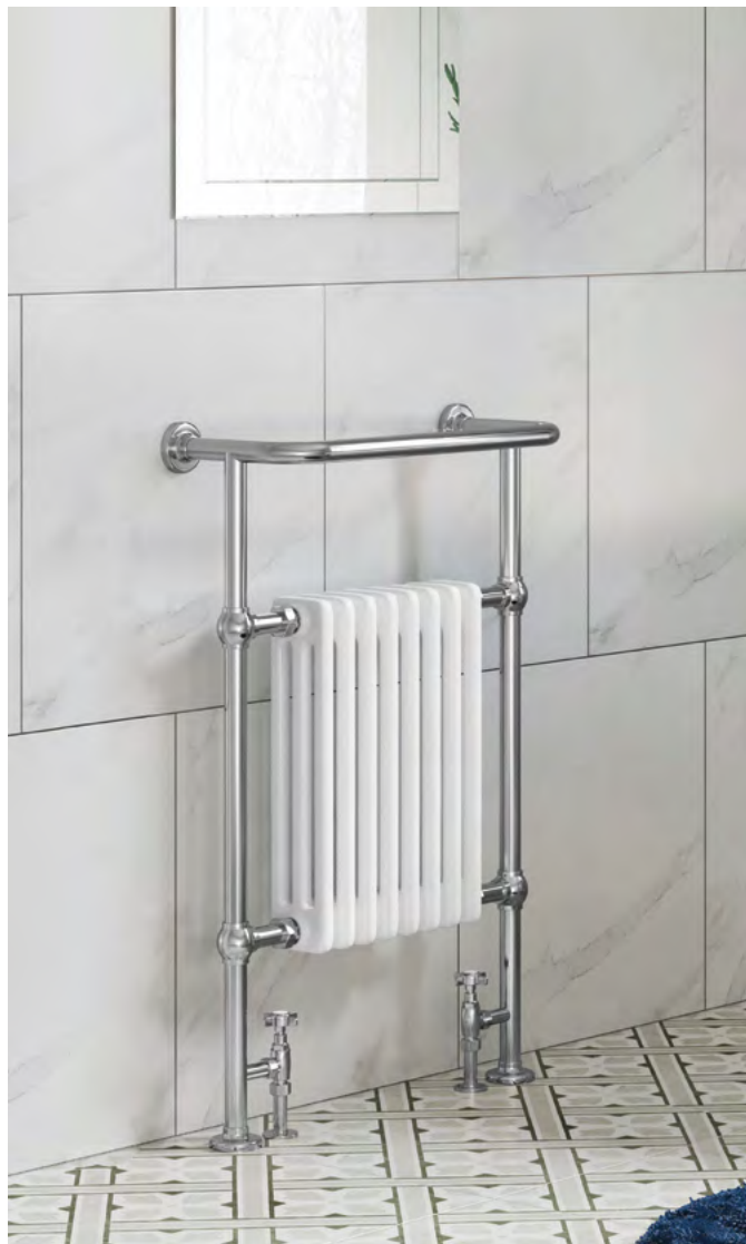
Floor mounted, must use angled valves
